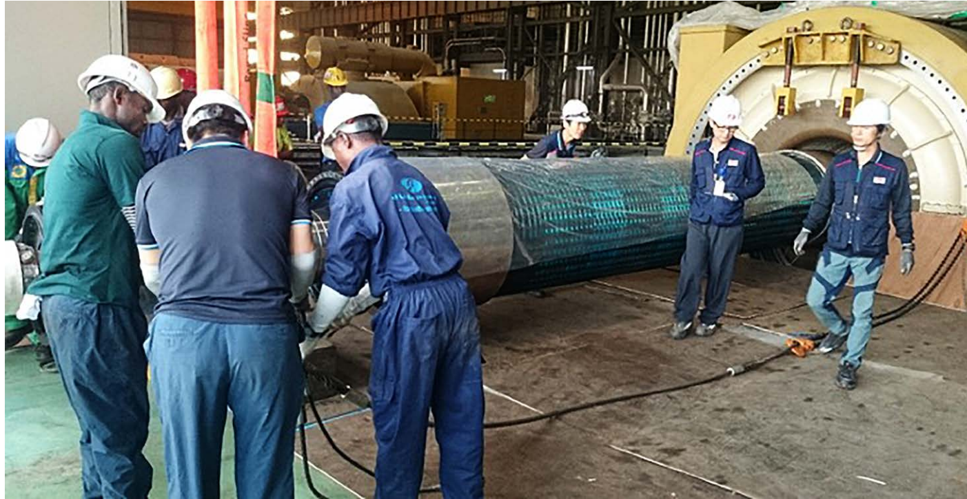
Unit 4 Genertor Rotor During Major Overhaul
