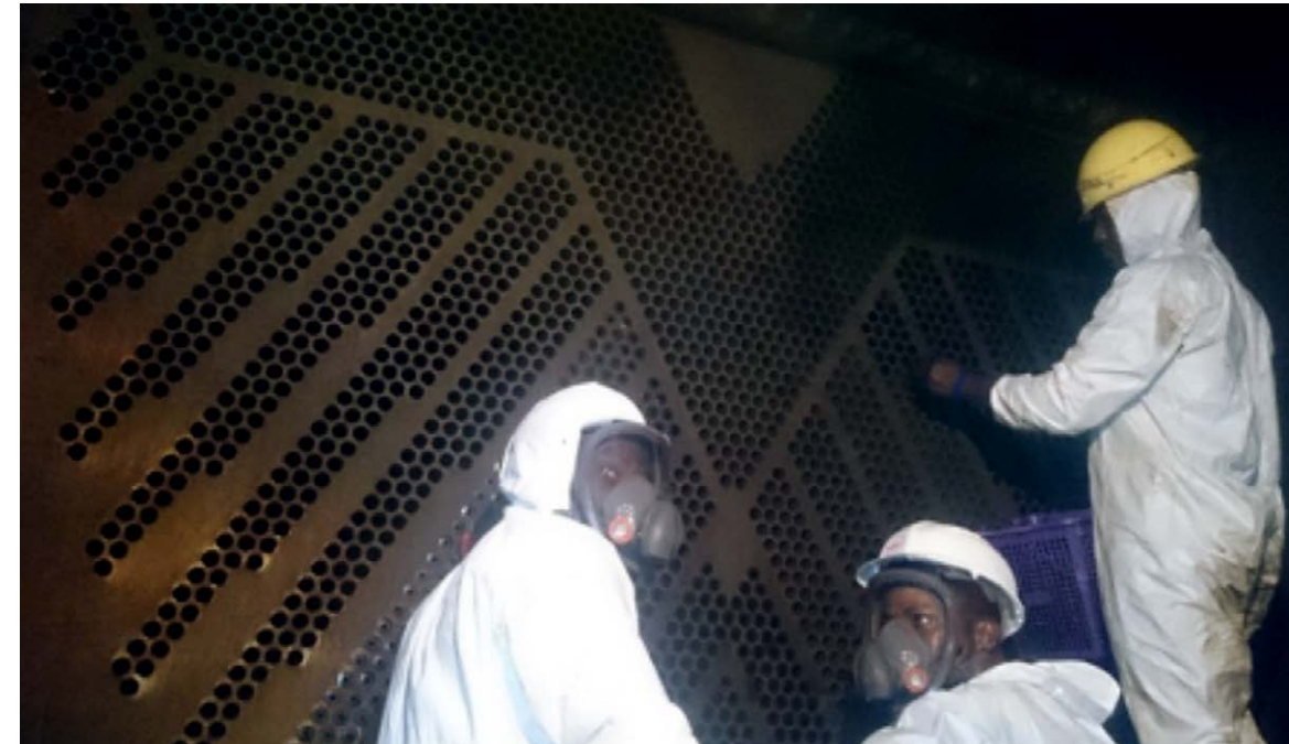
Maintenance Engineers during a condenser cleaning process
