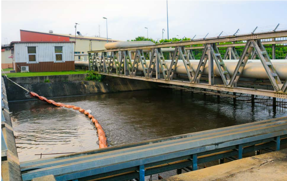
Floating Boom to mop up any oil on the discharge water
