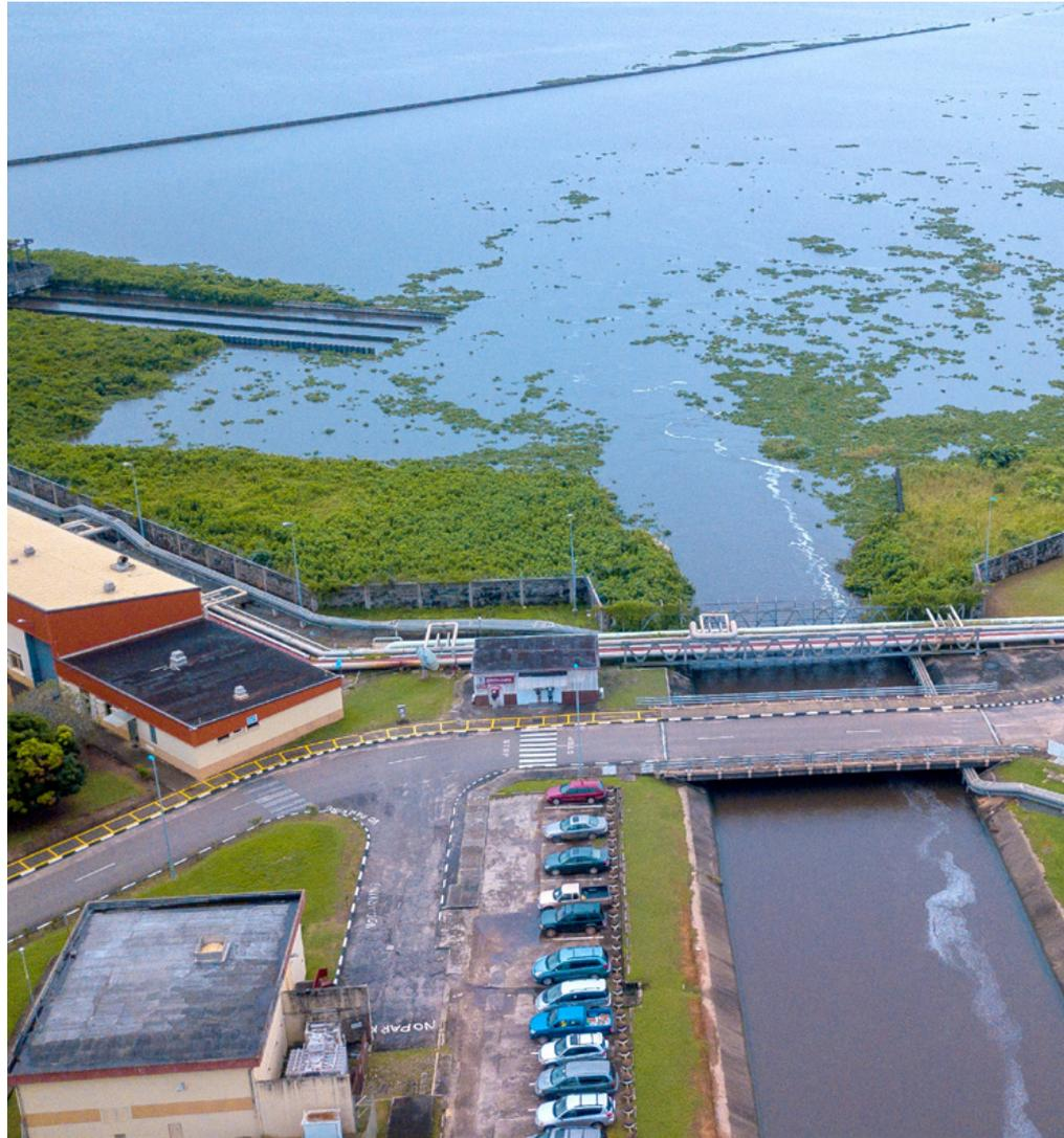
and width of the discharge canal ensures that the discharge water travels a long distance in order to dissipate substantial amount of heat before it eventually mixes with the larger water body. The quality of water has a lot of advantages on the process and environmental impact on the body of water (lagoon) for preservation of aquatic life and pollution free water that could affect communities living around the power plant.
